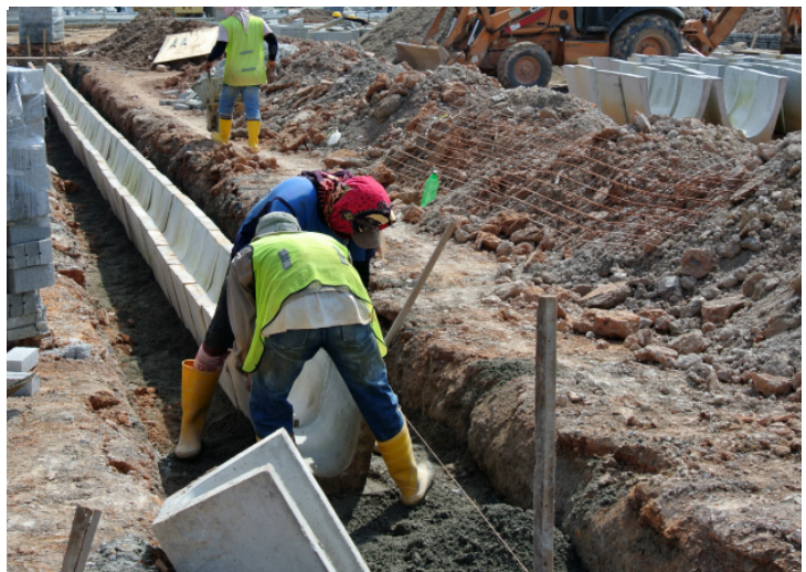
Workers install a V trench to direct runoff
